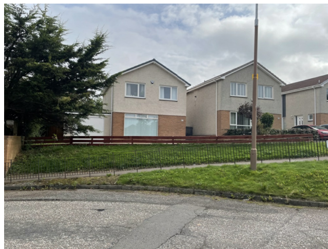
Existing Fence - Image 01 from Road North Bughtlin Road
